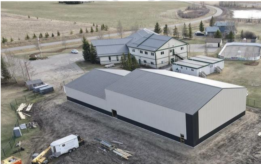
Aerial View of School Building and Expansion – May 2022
